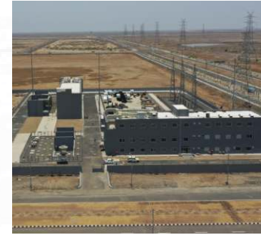
Power Substations 2 Substations (33/66 kv and 220 kv GIS) by Torrent Power
