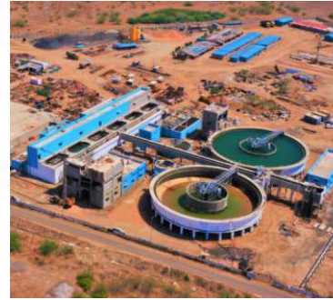
Water Treatment Plant 50 MLD Commissioned, expandable up to 150 MLD
