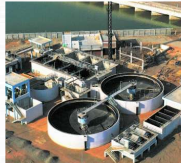
Sewerage Treatment Plant 10 MLD Commissioned, expandable upto 30 MLD
