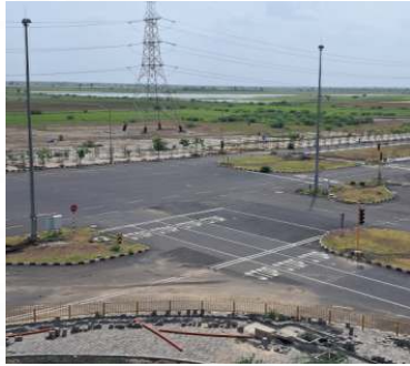
Internal Road Network 70 km Long, 18 to 70 m Wide
